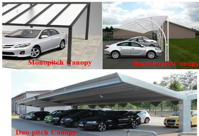
Fig. 1. Design of various carport canopies roof structures
